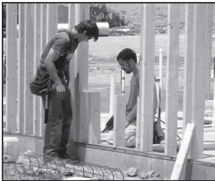
Volunteers were instrumental in building the new respite center in Hagerhill.
